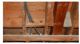
Electrical flex conduit needs fire caulking (red color) and the drilled hole in the blocking needs to be filled in.
