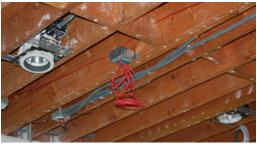
The red wire electrical box is for the smoke detector system. Notice the hole in the blocking through which the red wire passes which needs to be sealed.
